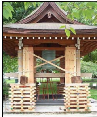
During renovation work on the Kobe Bell
